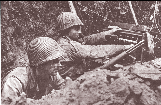
This fancy front-line switchboard is nerve center of communication for dug-in combat infantryman in France.
