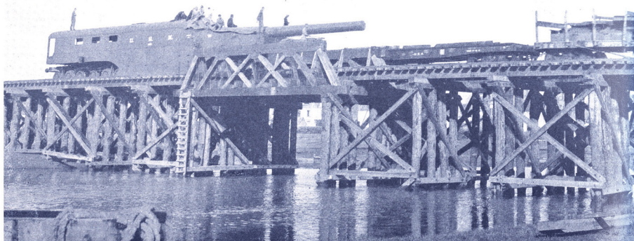
Trestles had to be strengthened to carry the immense weight—275 tons each—of the gun cars as they left St. Nazaire for the front.
